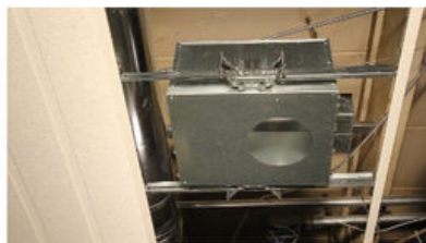
Fig. 70 Downlight suspension from T-bar
