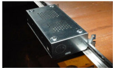
Fig.80 Mounted to T-Bar using the integral T-Wings
