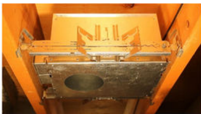
Fig. 69 Downlight suspension from wooden joists
