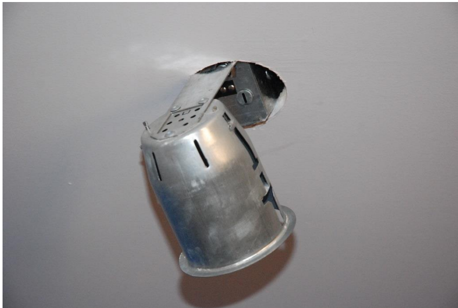
Fig. 7 Typical retrofit or remodeler assembly being rotated into hole in existing ceiling.
