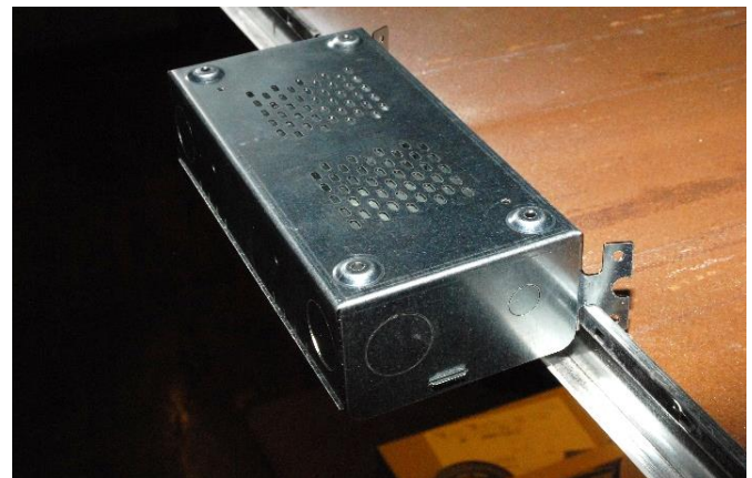
Mounted to T-Bar using the integral T-Wings
